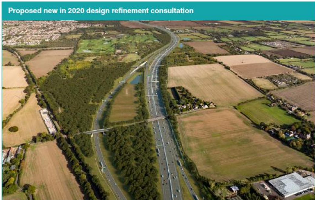
Figure 3-34. Design refinement consultation – proposed LTC/M25 junction, with new Ockendon Road bridge, looking north
