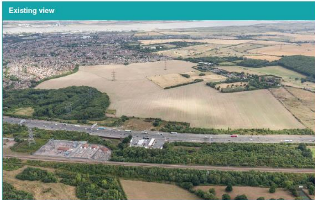
Figure 3-5. Existing A2, looking north
