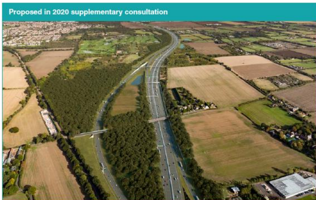
Figure 3-33. Supplementary consultation – proposed LTC/M25 junction, with new Ockendon Road bridge, looking north
