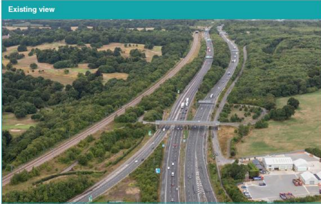
Figure 3-1. Existing M2/A2 along the A2 near Park Pale bridge, looking west
