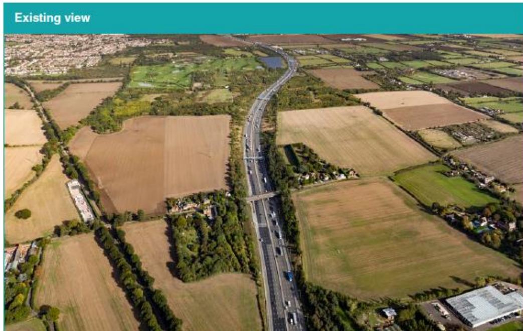
Figure 3-32. Existing M25 and Ockendon Road, looking north
