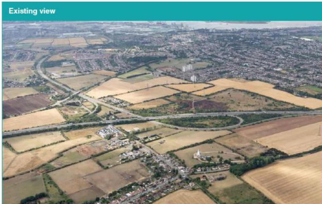
Figure 3-23. Existing A13/A1089 junction, looking south
