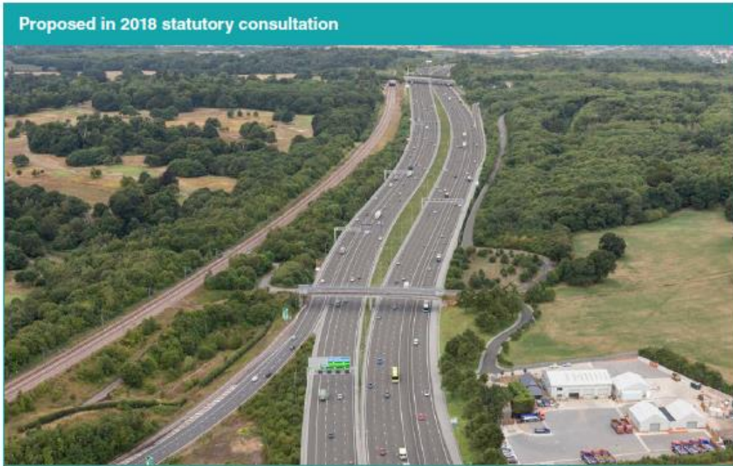
Figure 3-2. Statutory consultation – proposed M2/A2 along the A2 near Park Pale bridge, looking west
