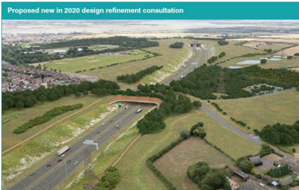
Figure 3-15. Design refinement consultation – proposed Thong Lane green bridge linking Gravesend and Thong and the approach to the southern tunnel entrance, looking north
